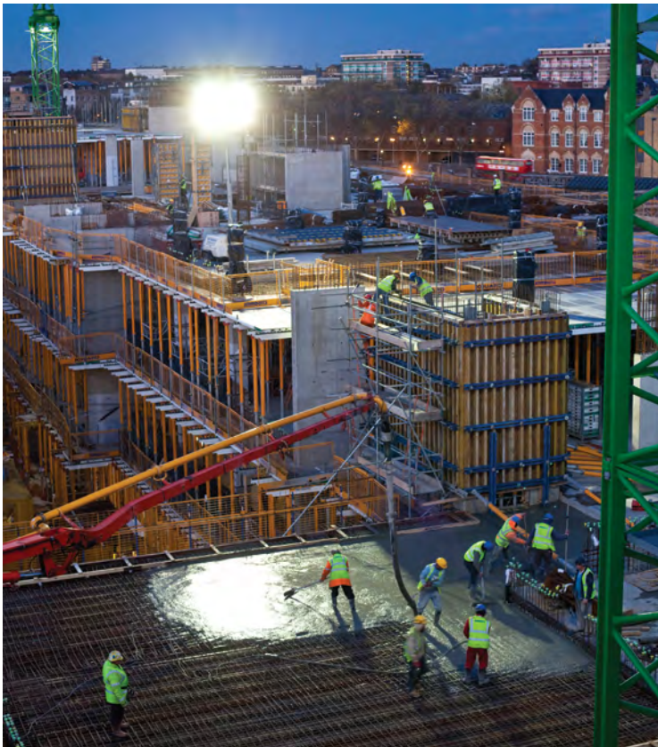
Pouring of the third floor southern studio concrete slab
