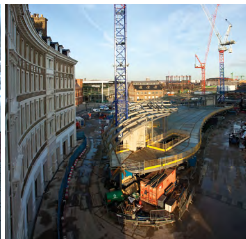
View looking north from the Great Northern Hotel façade
