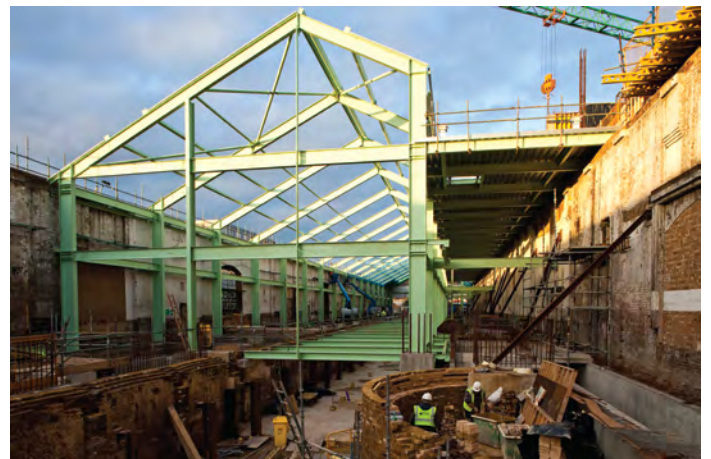
Steel portal frame within the Western Transit Shed
