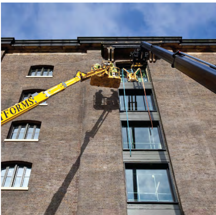
Installing the new glazing to the Granary façade
